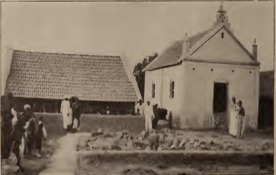
A TYPICAL VILLAGE CHURCH AND SCHOOL BUILDING, WITH TEACHER'S HOUSE, PULIKURICHI, SOUTH INDIA
